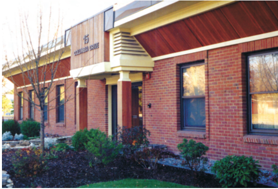
Monarch International's 30,000 square-foot facility in Amherst, New Hampshire, U.S.A.
